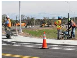
Workers race to finish up the Matanzas Woods Parkway-Interstate 95 interchange project last week, with the ramp to southbound I-95 visible in the background. The on-off ramps are scheduled to open Monday afternoon following a ribbon-cutting ceremony. NEWS-JOURNAL/DAVID TUCKER
